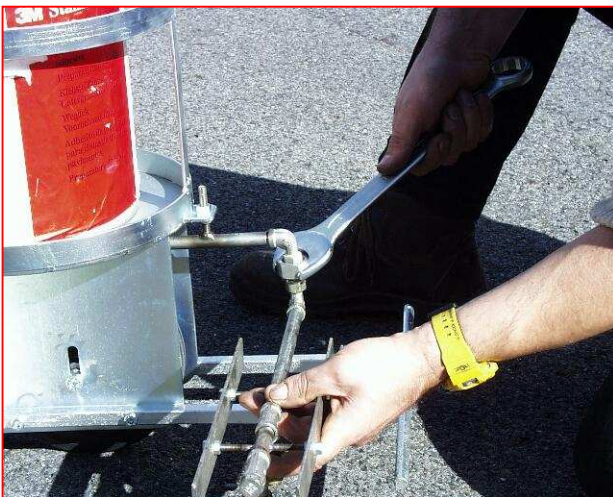
Figure 3: Tighten Main Screw
