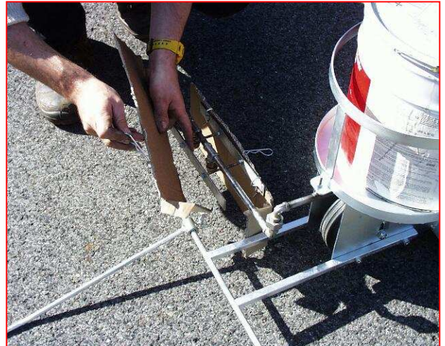
Figure 5: Add protective cardboard
